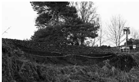
Above and Above Right: The landslide in December 2015
