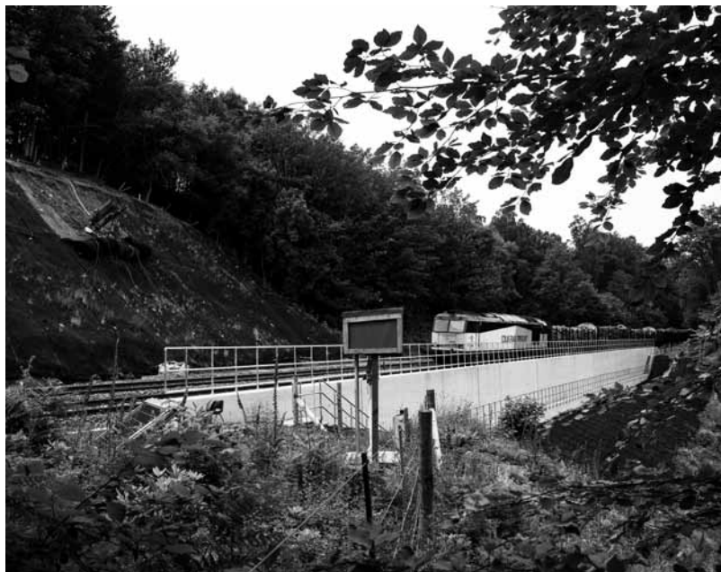
660026 hauls the log train over the new structure at Eden Brows on 21st June.
